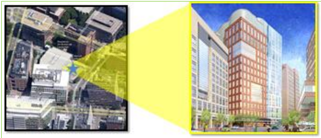
Figure 1: A look at the location of 75 Ames Street in Cambridge (courtesy of ELKUS|MANFREDI ARCHITECTS)
